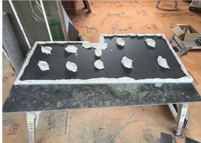
Dot-and-dab adhesive pattern with continuous edge coverage
