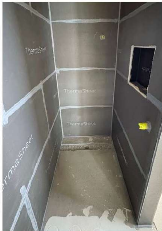
Joint treatment to a ThermaSheet-lined shower area
