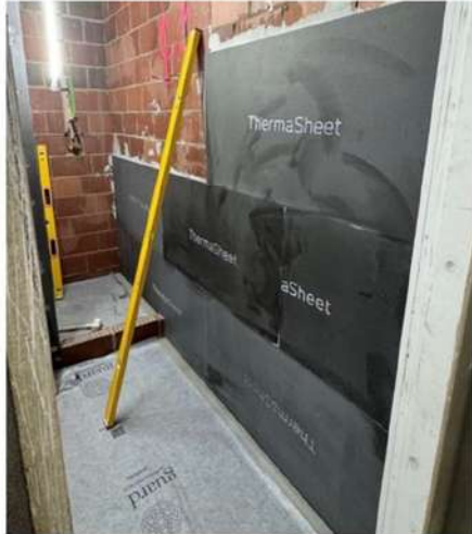
Boards installed to masonry wall
