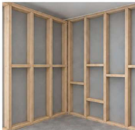
Timber stud wall prior to fixing Thermasheet
